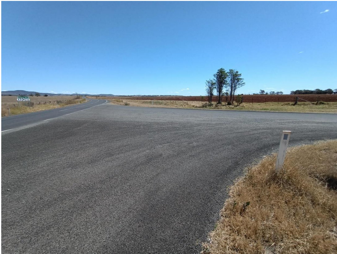
Image 1: Bunya Highway / Mannuem Road Intersection Looking South-West
