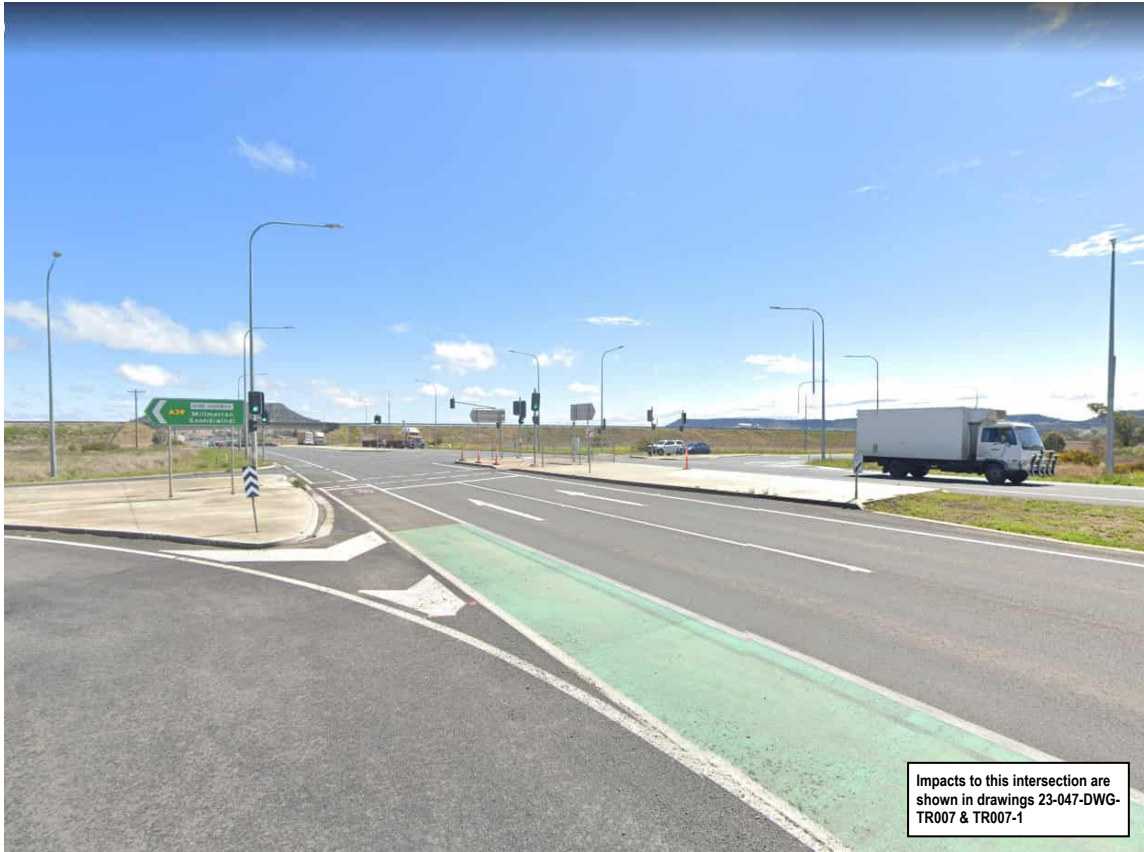
Image 7: Toowoomba Bypass / Warrego Highway Intersection (Location 7) Looking North-West
