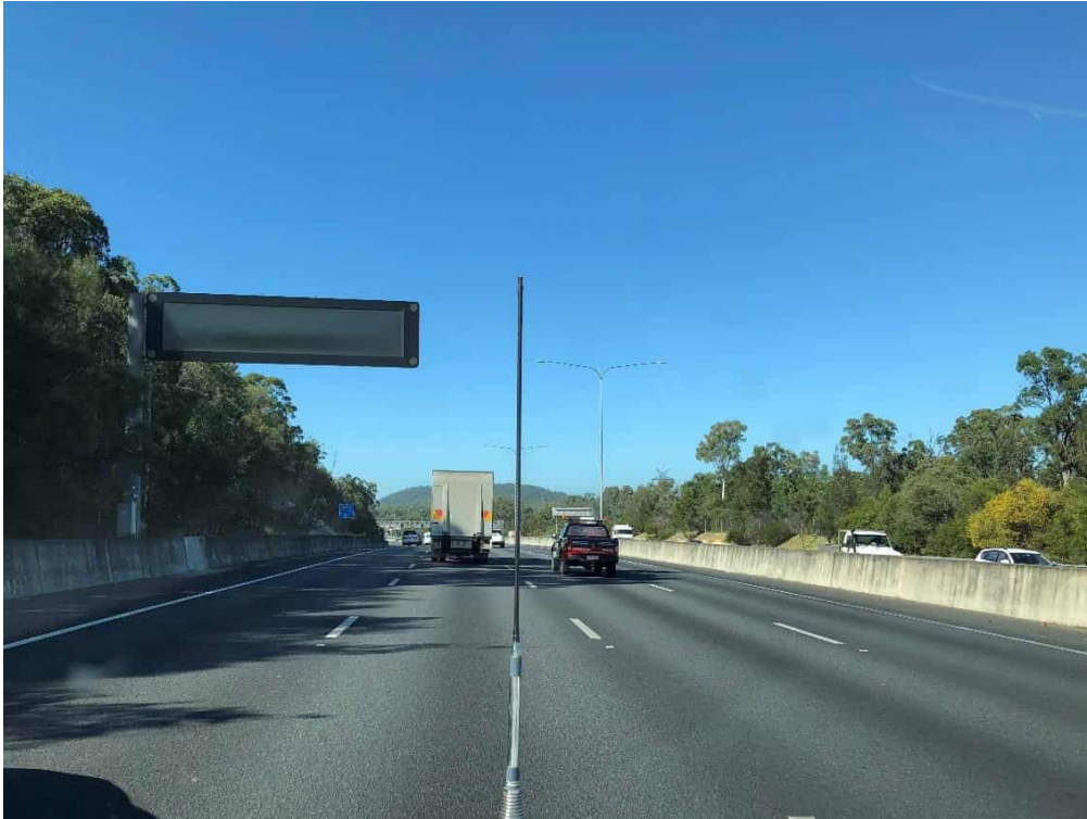
Image 5: Example Overhead electronic sign structures on Gateway Motorway
