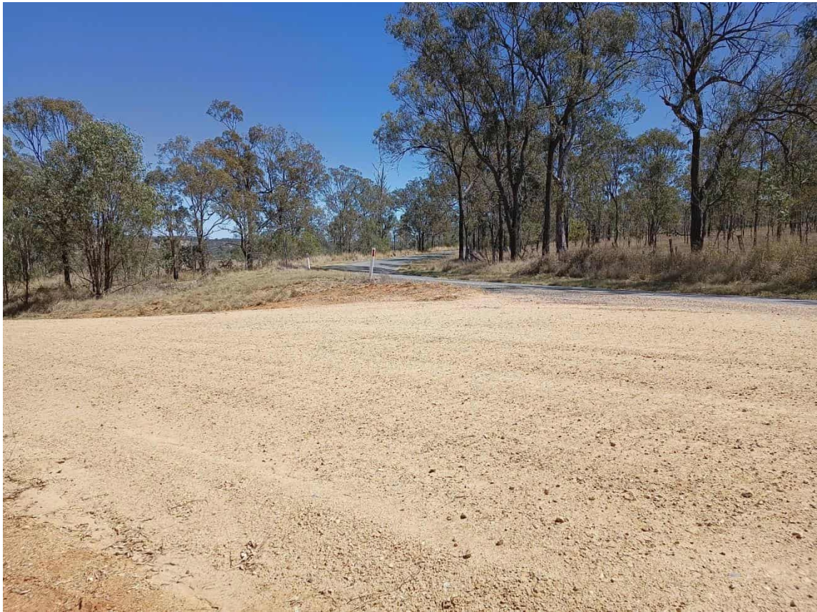
Image 5: Nords Road / Red Tank Road Intersection Looking North-West
