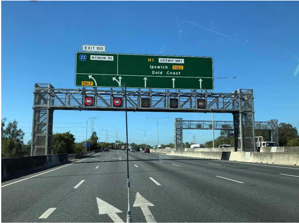
Image 4: Example Overhead Structures on Gateway Motorway
